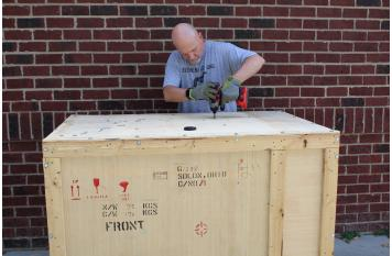
6. With the drill and 10mm socket, remove the lag screws from the top of the crate.
